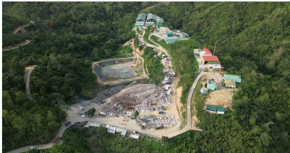
Solid Waste Management Centre, Tuirial
