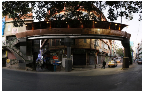
Pedestrian Overbridge at Bazar Bungkawn
