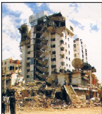
Fig. 3.3a: Destruction caused by an Earthquake in Gujarat
