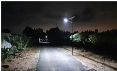
PROVIDING STREET LIGHT
