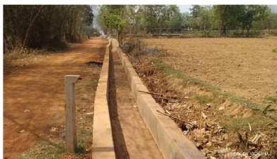
PROVIDING DRAINAGE SYSTEM
