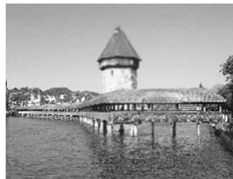
The Chapel Bridge
